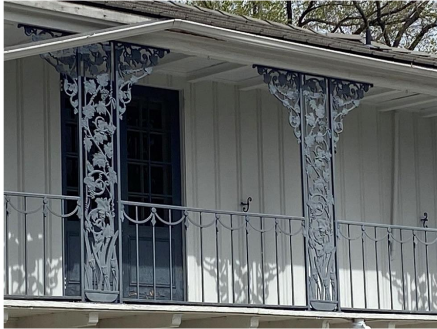
Figure 3 – Ornamental iron work on the balcony of the Luella Garvey House. Photograph by Alicia Barber.
