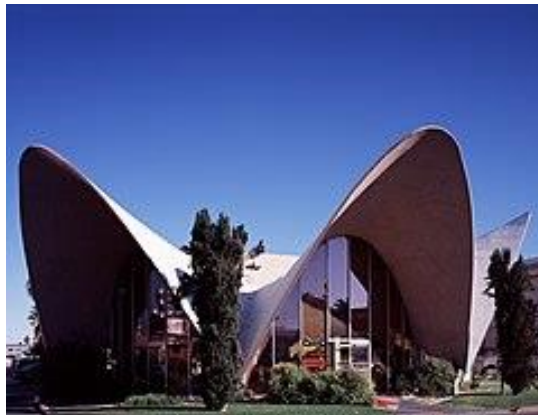
La Concha Motel, front lobby view, 1961
